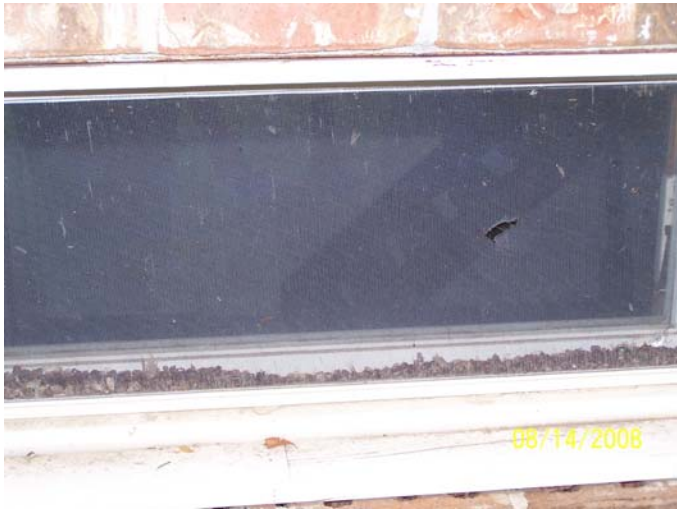
Basement window – Clean and caulk
