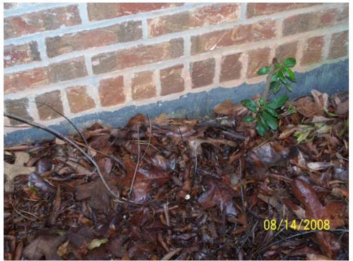
Grading at foundation. Increase and remove debris
