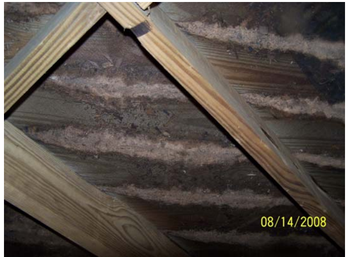
Netting under screened porch. Retains water
