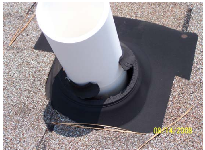
Replace vent boots on all three plumbing vents
